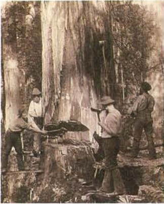
Adventure Bay sawmill, Tasmania. The axeman wears moleskin trousers (here held up with a belt, as braces restricted the movement of the shoulders), bowyangs, a slouch felt hat, a flannel undershirt and cotton topshirt and a pair of strong boots, studded to prevent slipping. Axemen used a small whetstone to sharpen the edges of their blades, and lengths of strong string or copper wire to repair a split handle. Sometimes, as in this picture, a crosscut saw was used. Thus dressed and equipped, the best axemen could work for eight or ten hours a day through most kinds of weather.
